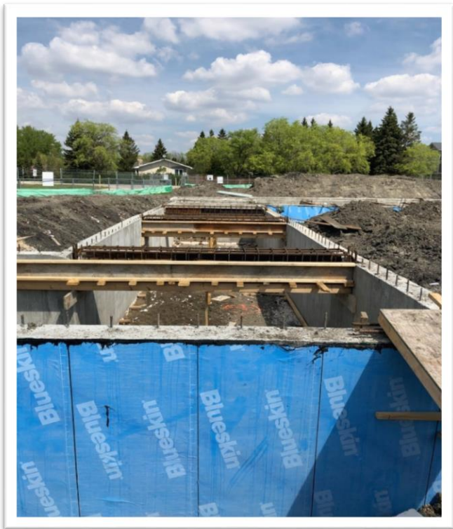
Weatherproofing foundation wall with Blueskin
