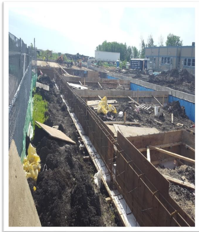
Framing footing wall North side classrooms
