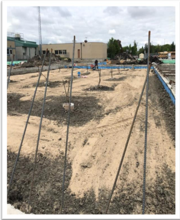
Gym area floor prepared for concrete pour
